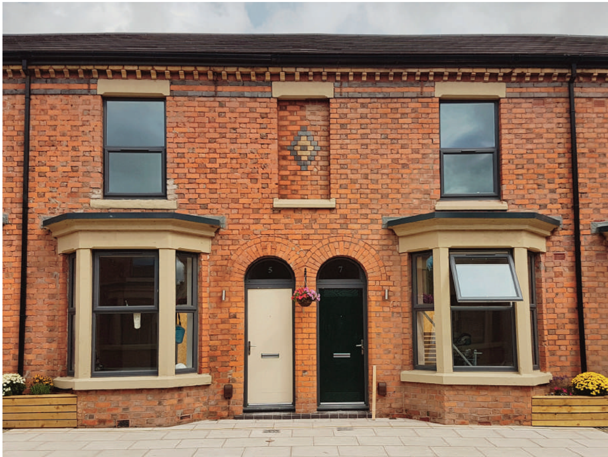
2017: Newly refurbished and adapted houses on Voelas Street, in the Welsh Streets
