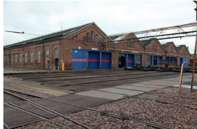
Railway works in the Wolverton Conservation Area
