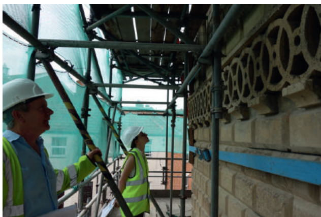
Inspecting progress from the scaffold at Castle House
