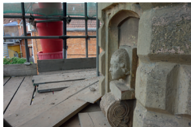
Concrete decoration on the façade
