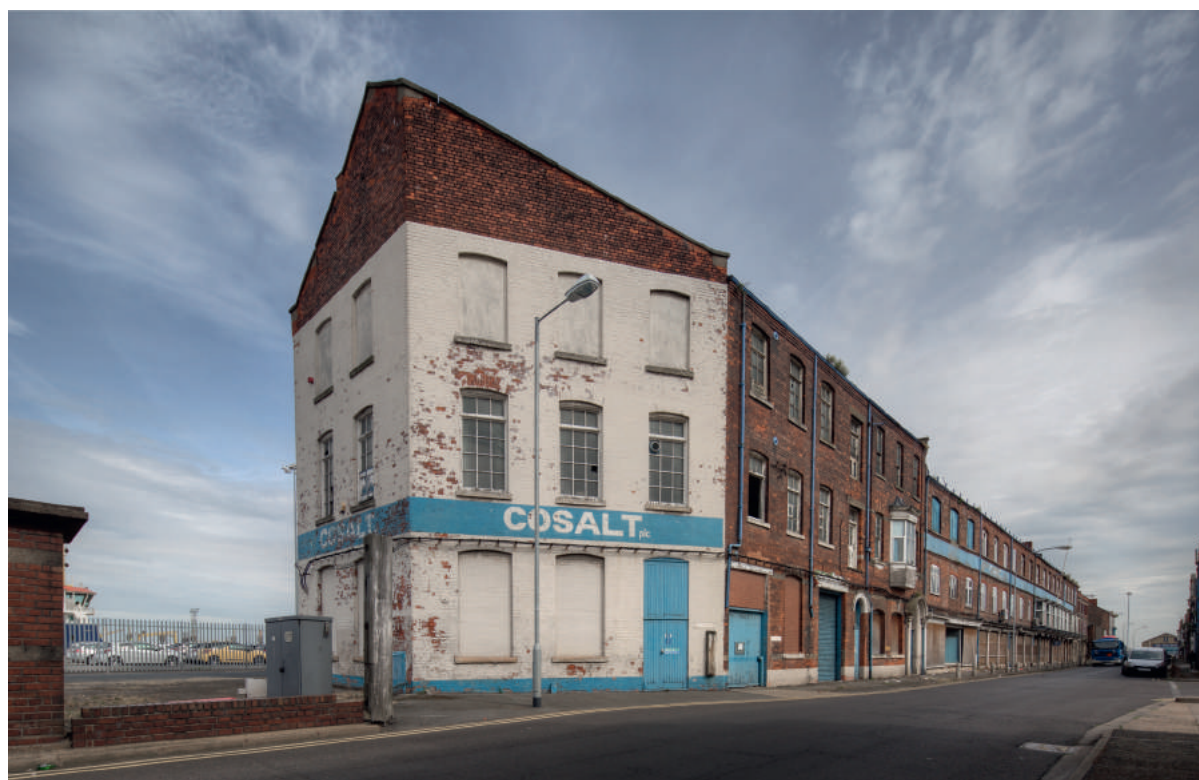
The Cosalt buildings on Fish Dock Road, subject of a major SAVE campaign in 2016. Image: Eveleigh Photography
