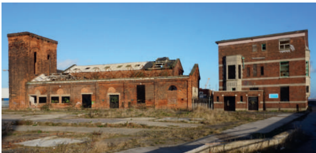
The Pump House at St Andrews Dock, Grade II listed. Image: Ian S, Geograph
