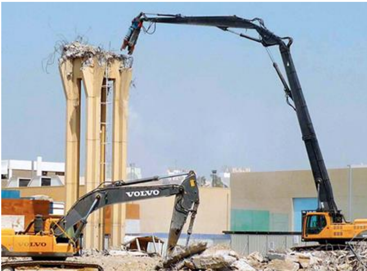
Photograph 6: High level Plant being used for demolition
