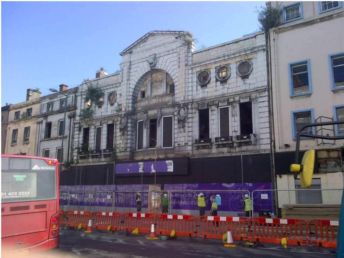
Photograph 5: The Futurist on 14 th May 2016 with scaffold largely removed
