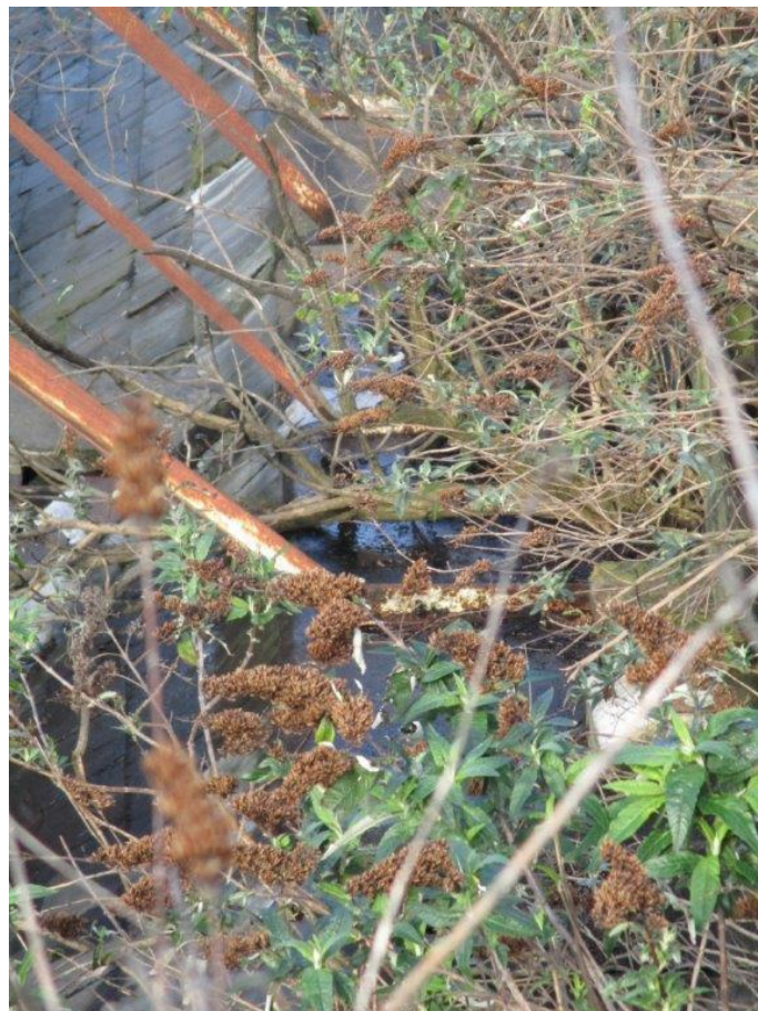
Photograph 6: Base of restraint straps
