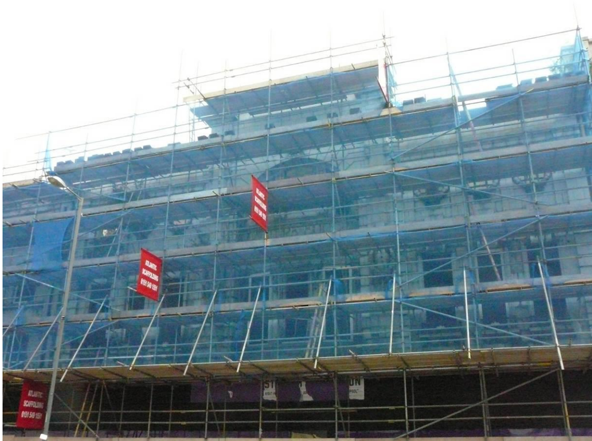
Photograph 4: The Futurist on 10 th May 2016 with scaffold erected
