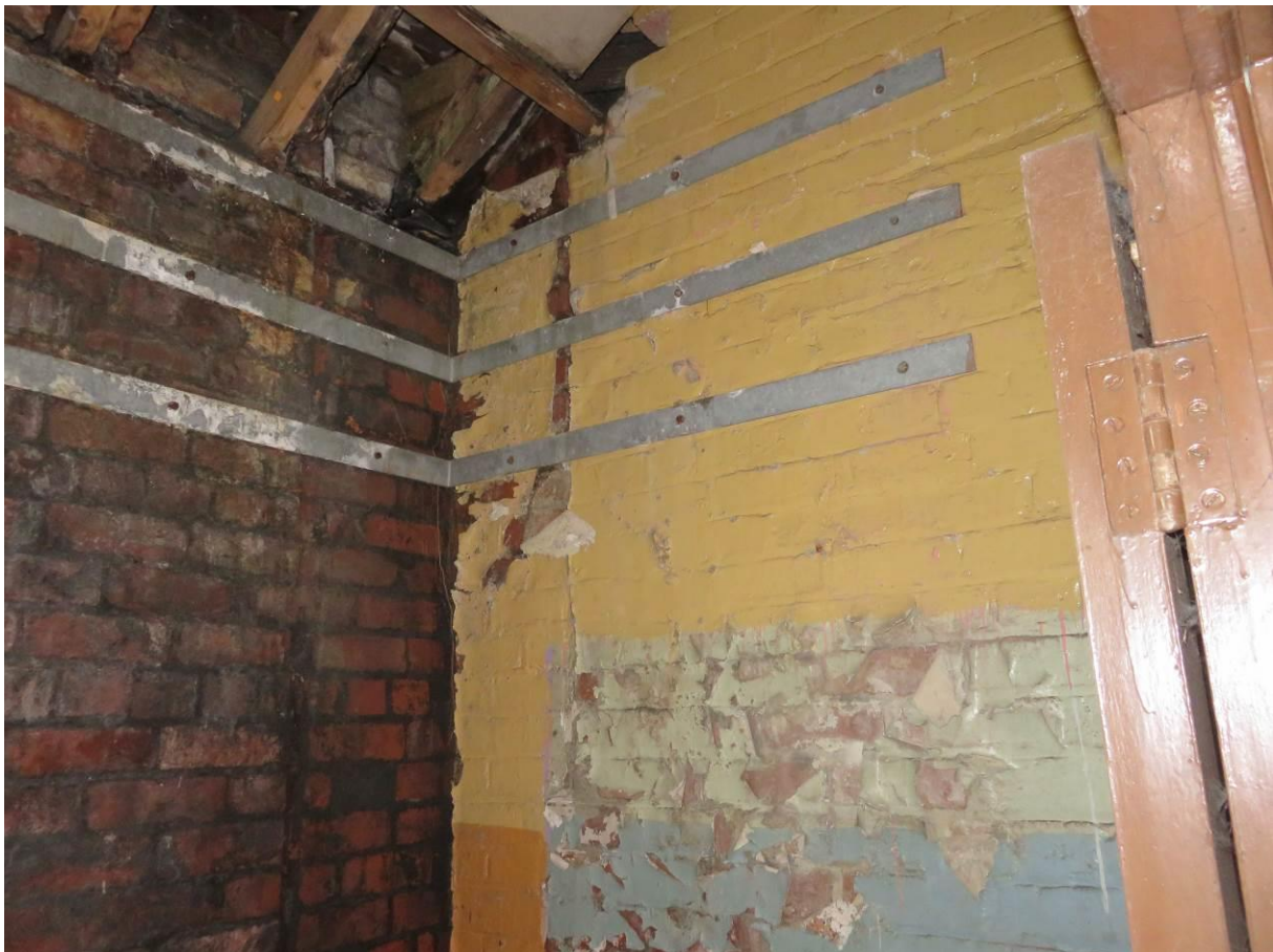
Photograph 2: Cross wall with temporary restraint straps
