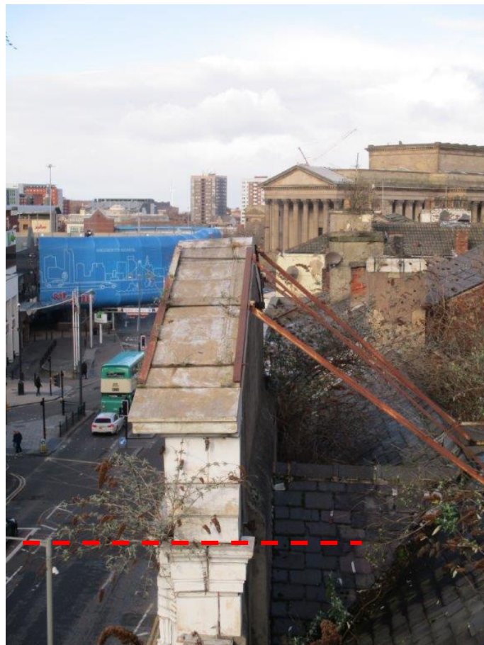
Photograph 8: Suggested position of dismantling
