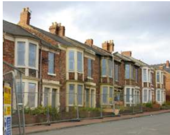
Condemned houses, now demolished, in Saltwell and Bensham, Gateshead
