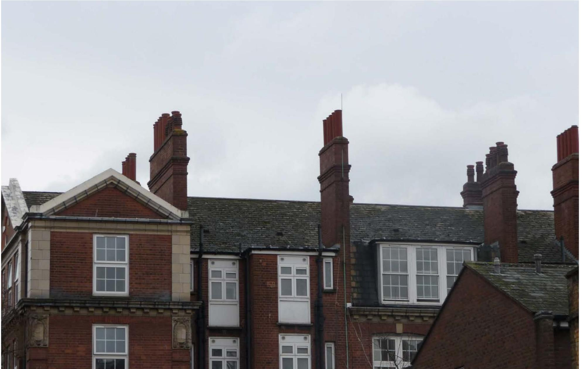
Slate hung mansard roof and original tall brick built chimneys, Block 'A', William Sutton Estate
