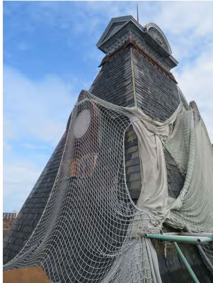
Photograph 80: Clock Tower roof structure
