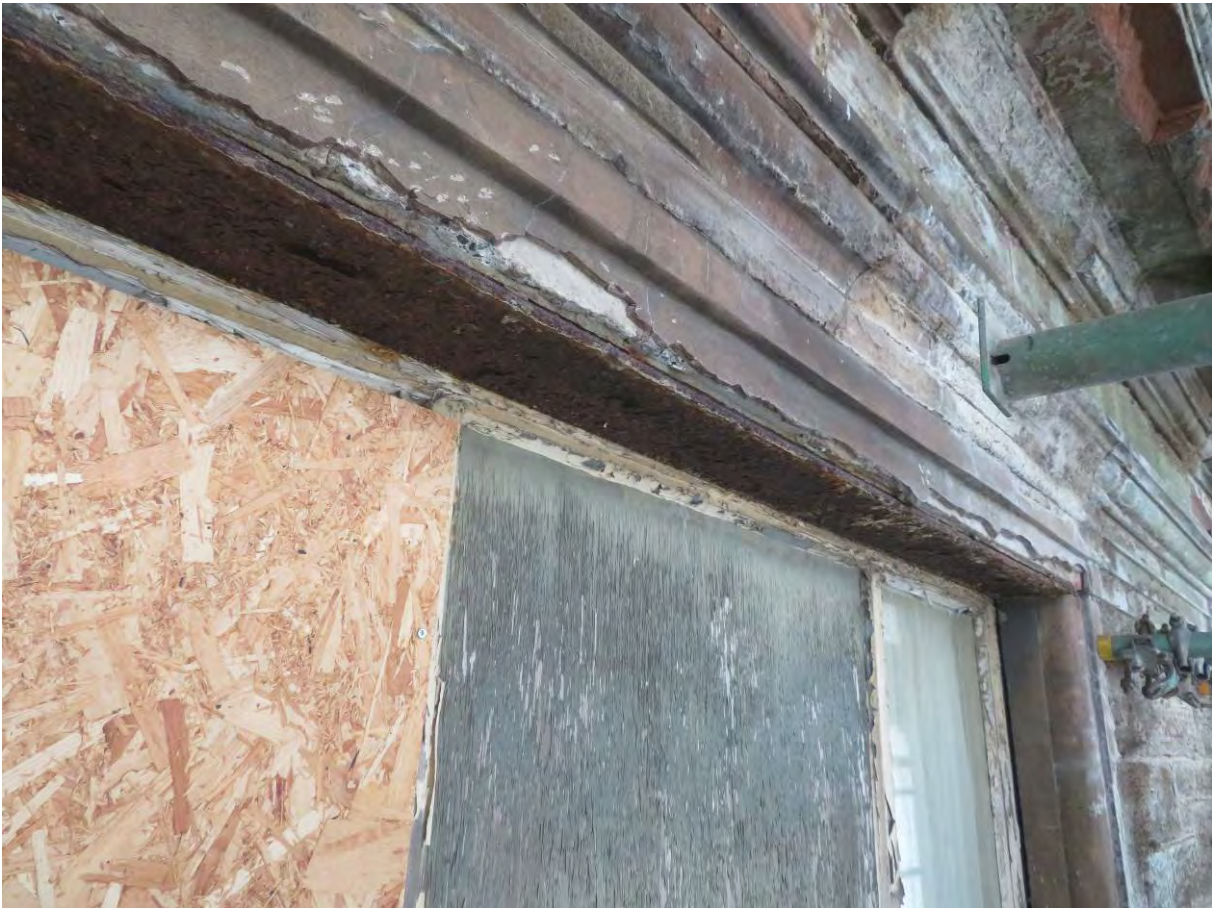
Photograph 51: Steel plate flat bar over window
