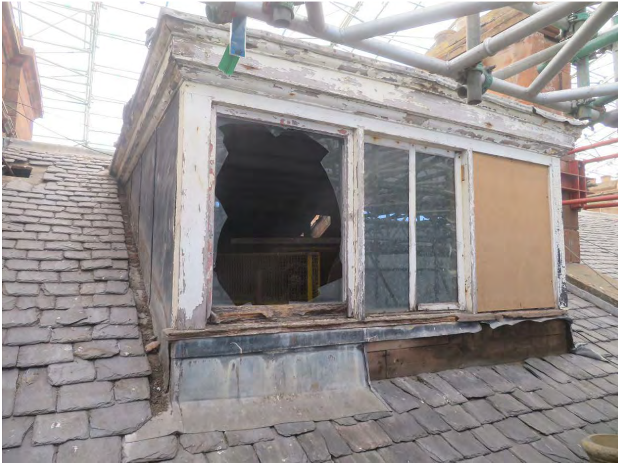
Photograph 31: Added dormer to the west elevation above lift area
