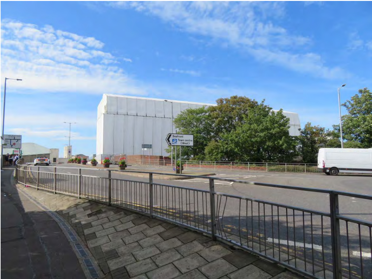
Photograph 7: South range east elevation
