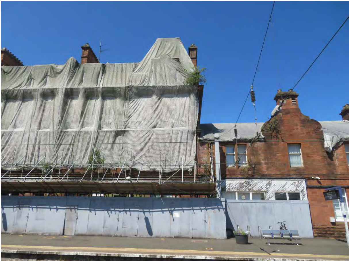
Photograph 93: Hoardings to lower section of east elevation to north range
