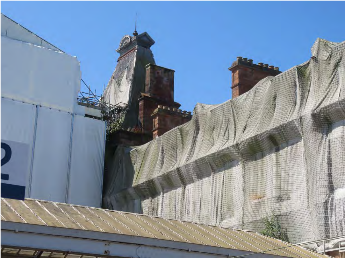
Photograph 92: Sheeting to east elevation of the North Range
