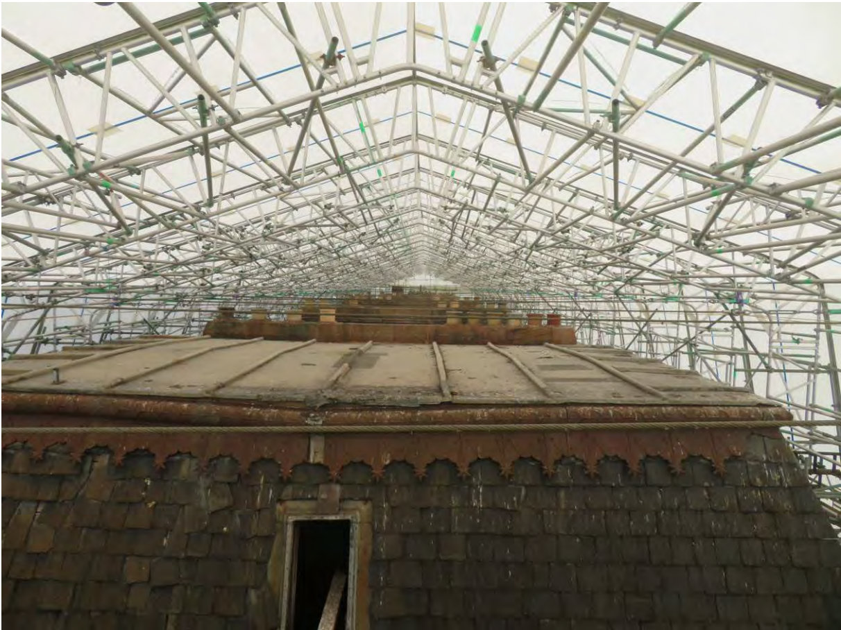
Photograph 9: High level scaffold as seen over South range
