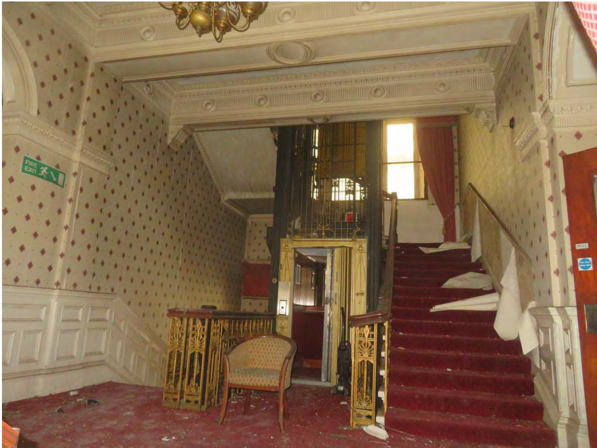
Photograph 79: Elevator and main stair at first floor level
