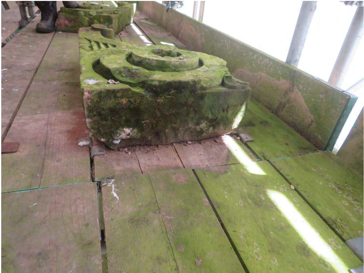
Photograph 15: Dismantled stones laying on scaffold
