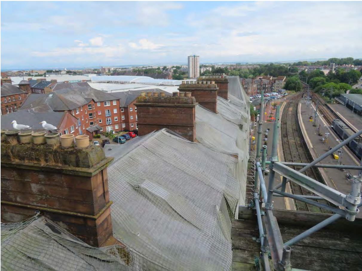
Photograph 91: Sheeting over North Range roof
