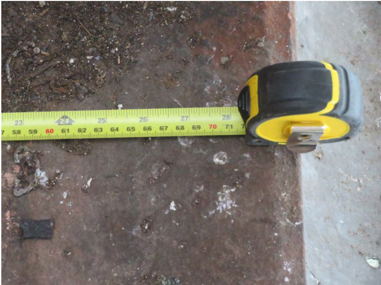
Photograph 29: Wall thickness at position where dormer exposed to east elevation
