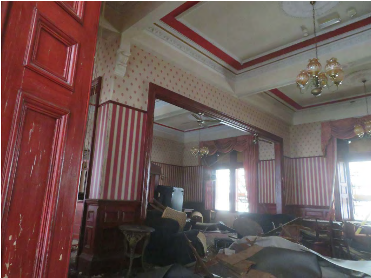
Photograph 77: Principal room with ceiling in reasonable condition
