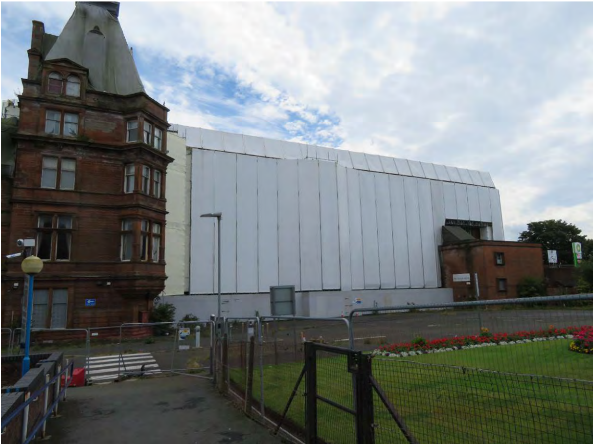
Photograph 5: South range west elevation with scaffold structure
