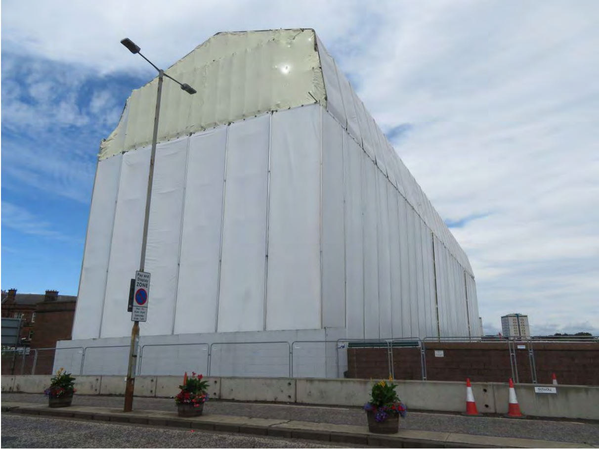
Photograph 6: South range, south and east elevation
