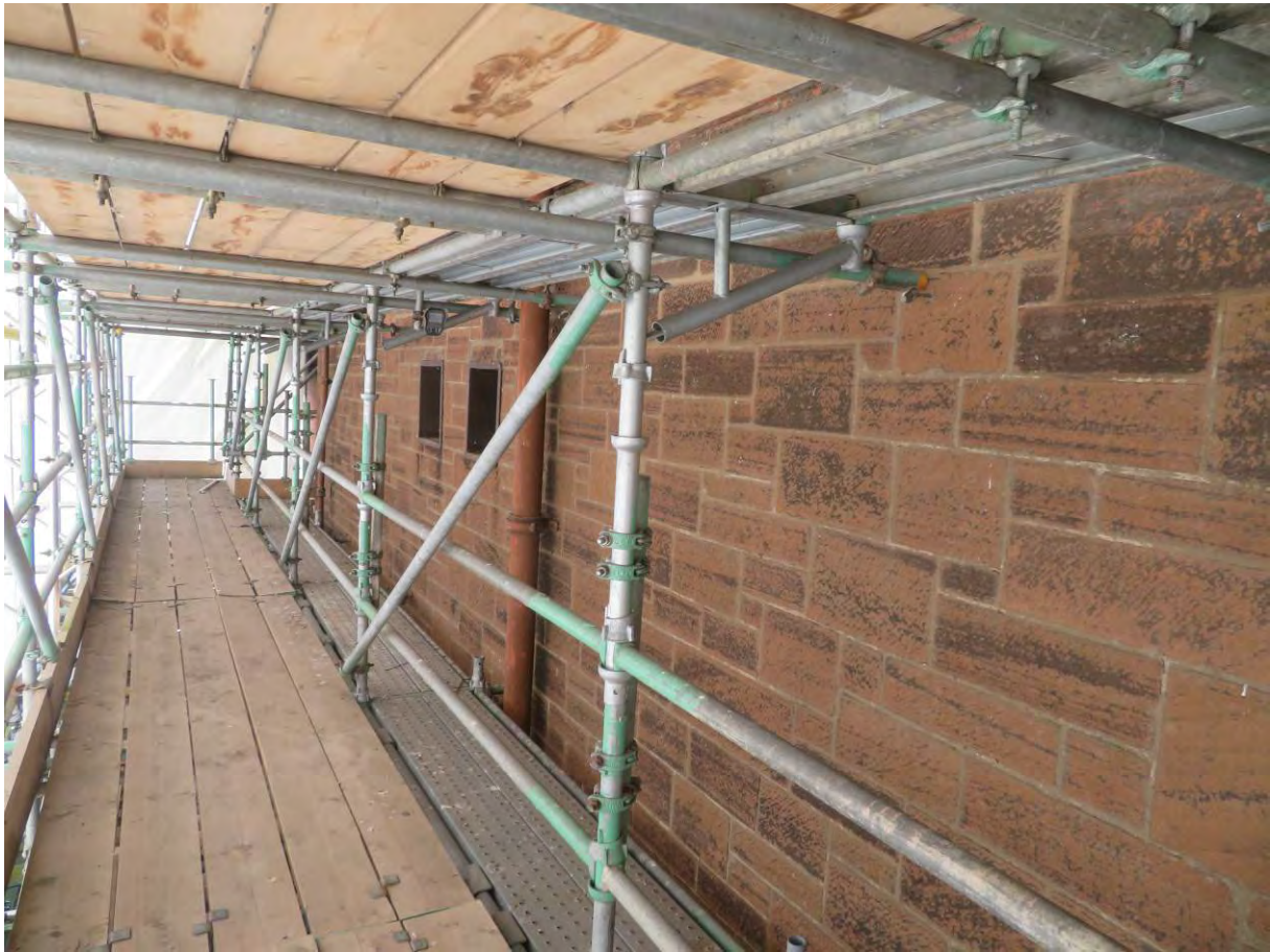
Photograph 63: Wider joints to track side elevations were less visible
