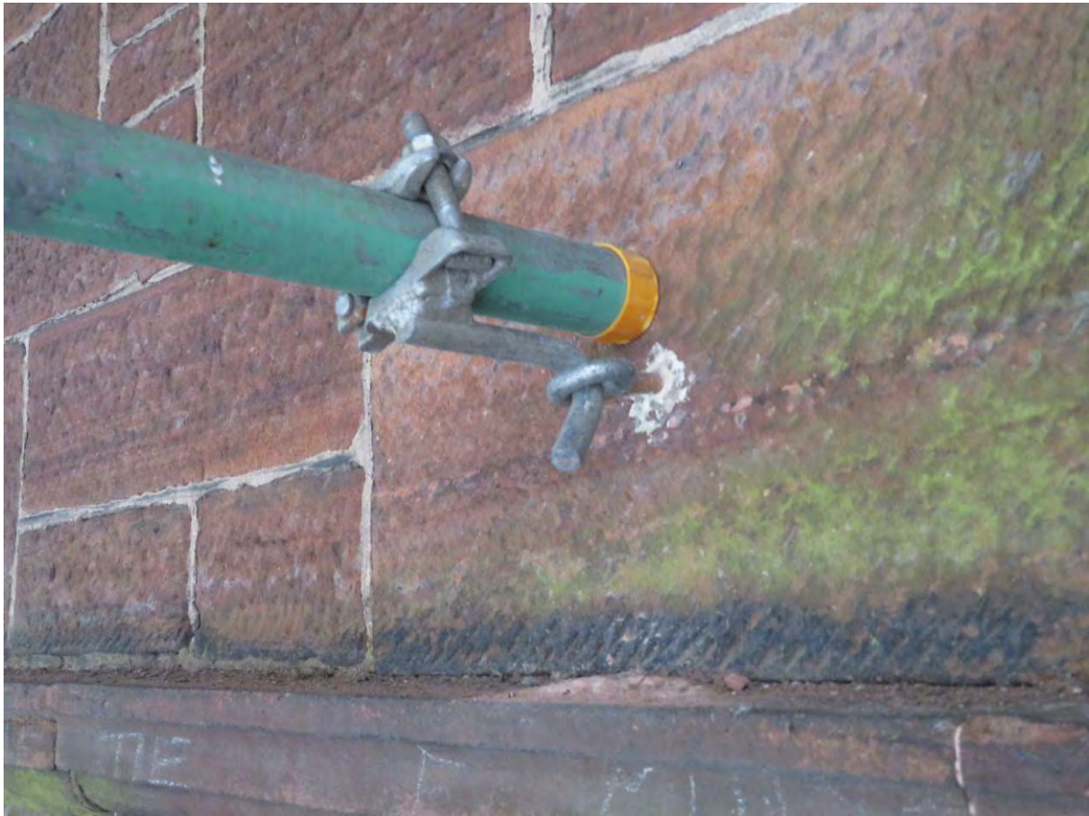
Photograph 11: Fixing into masonry from scaffold
