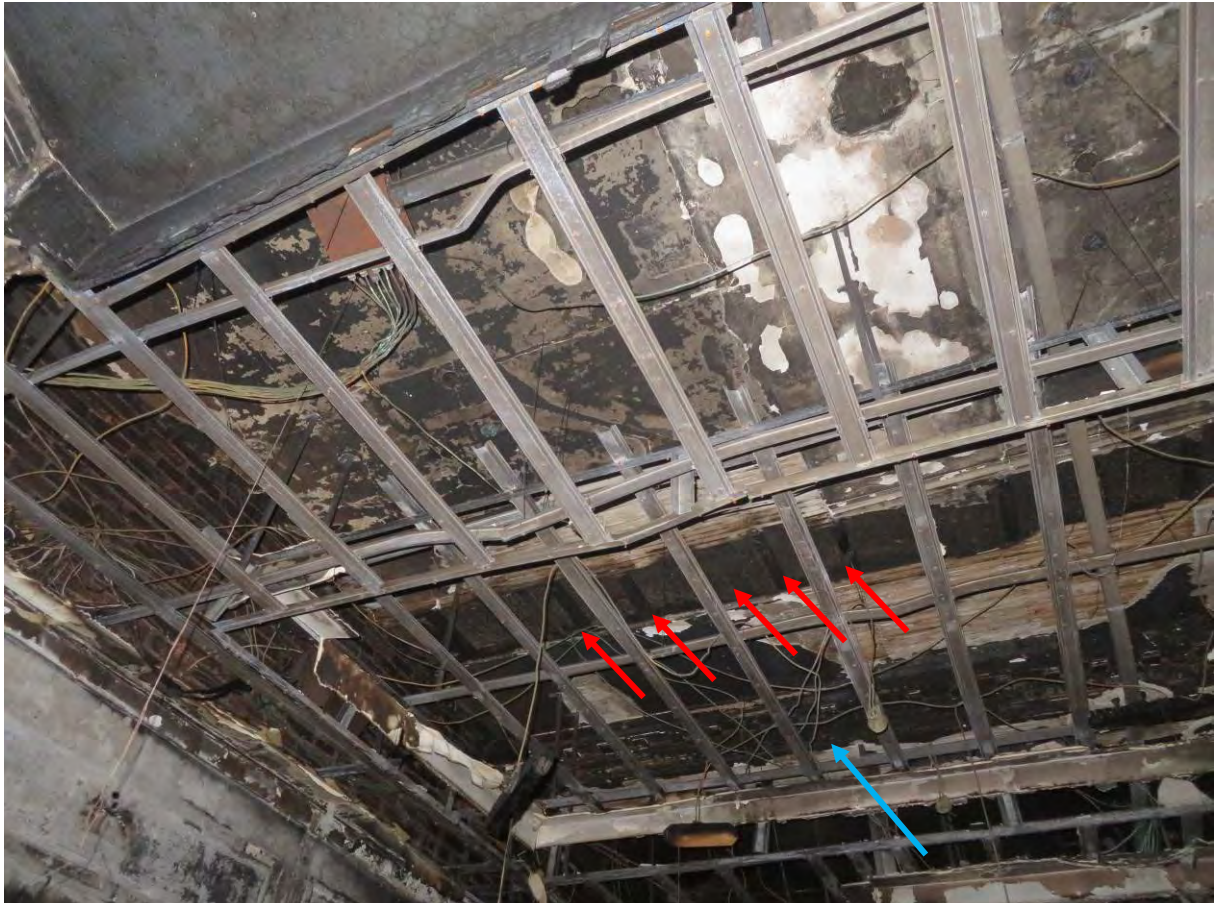
Photograph 78: Iron/steel beams (red) and concrete jack arches and main beams (blue)
