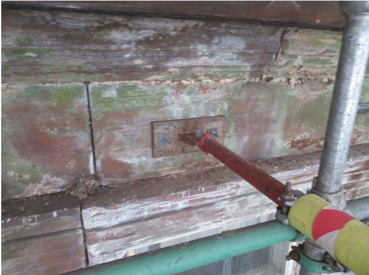
Photograph 12: Fixings into masonry from scaffold
