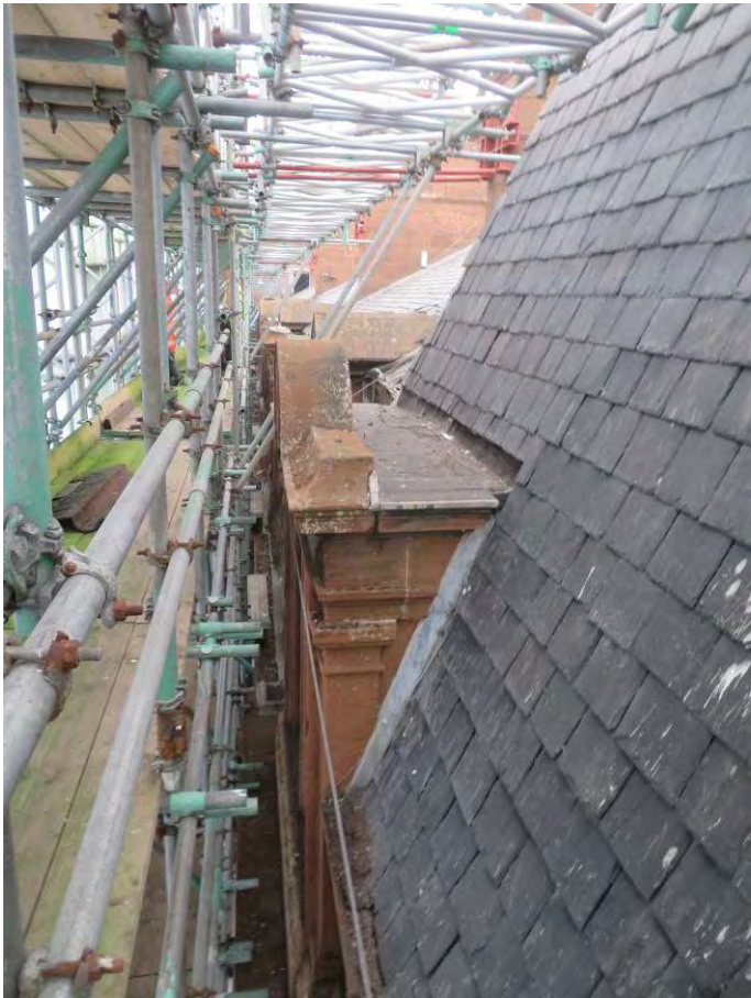
Photograph 25: Pedimented dormer to west elevation
