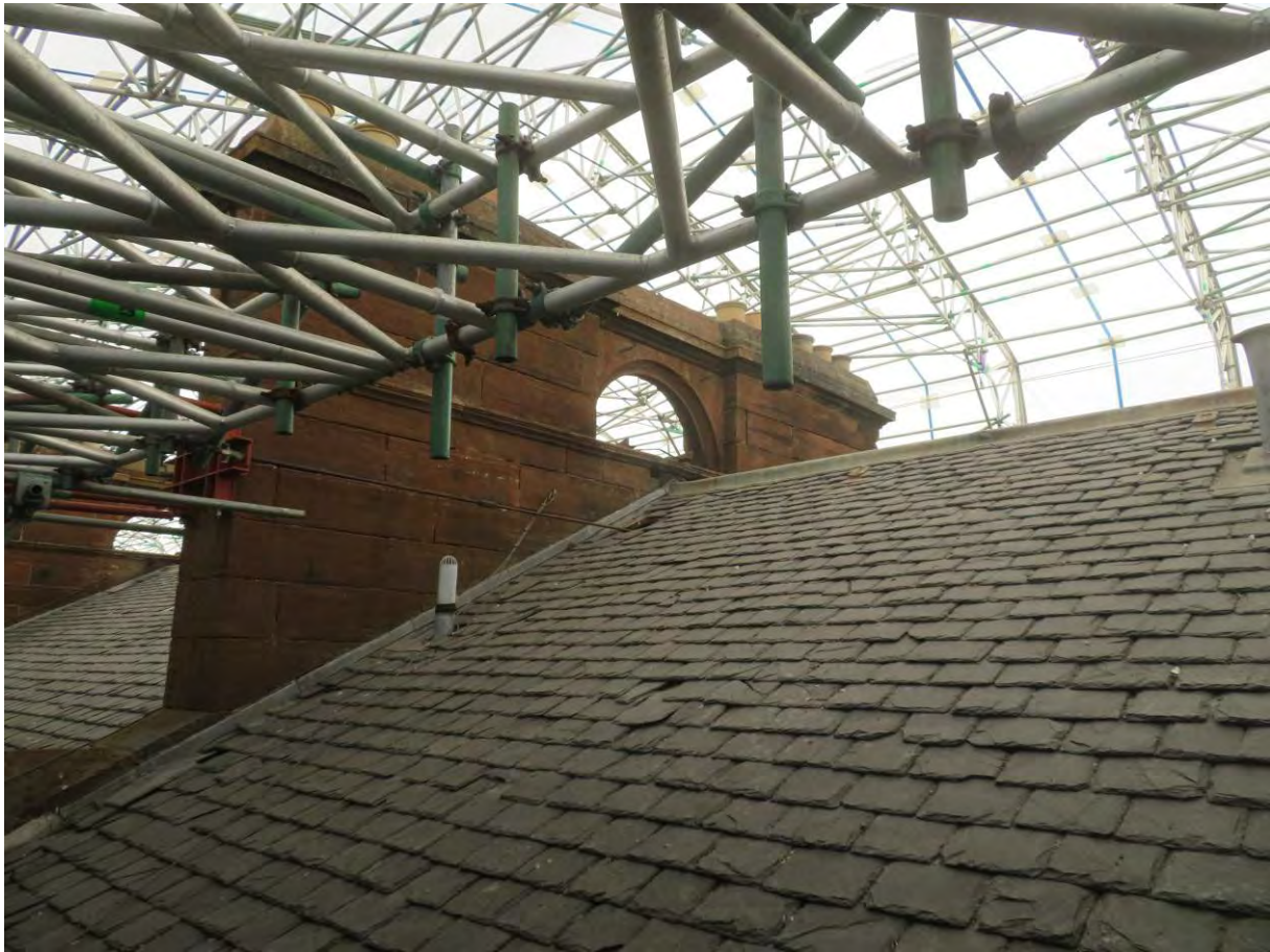
Photograph 17: Roof covering to south range west elevation
