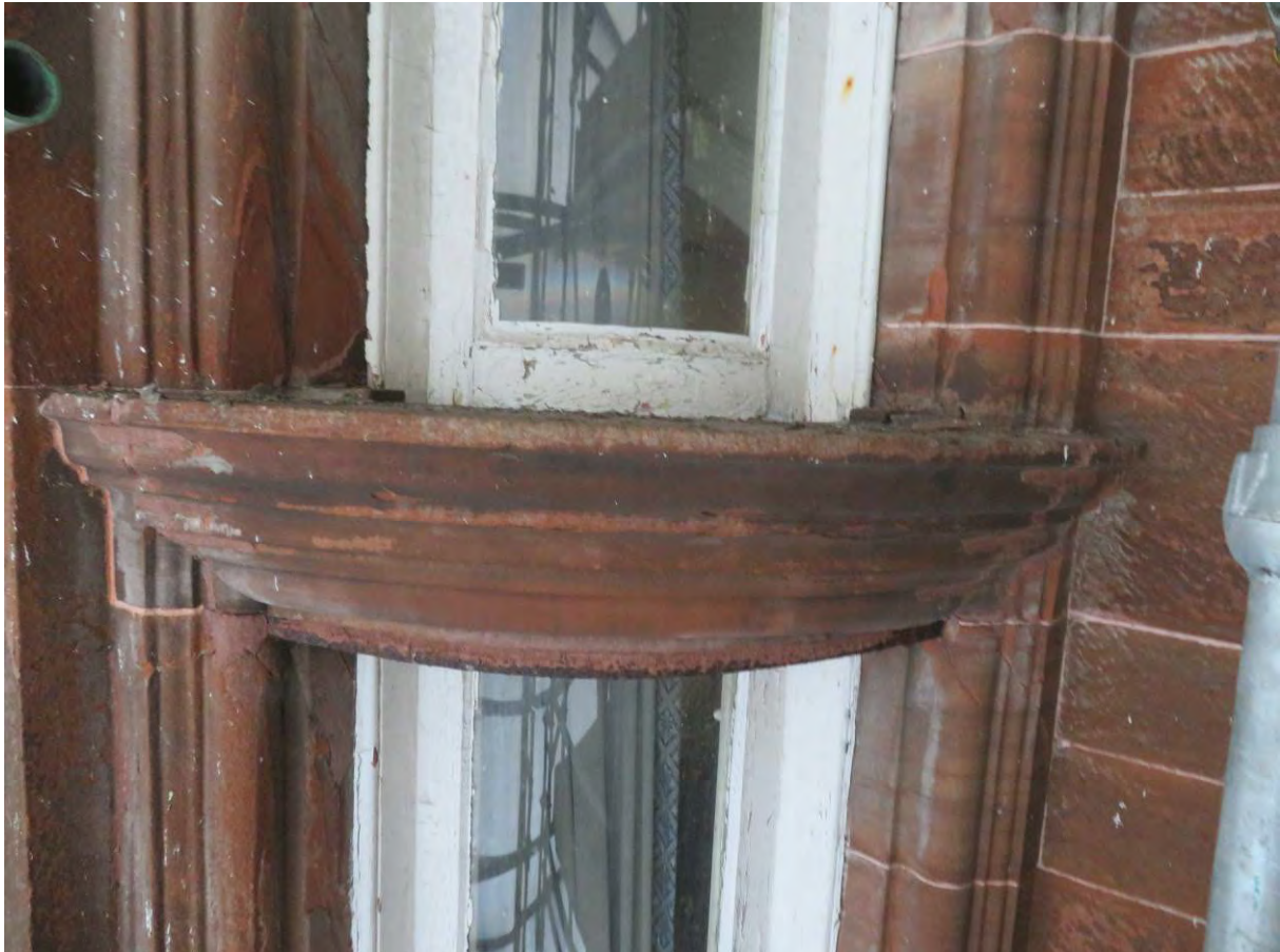
Photograph 64: Curved stone lintels and cured
