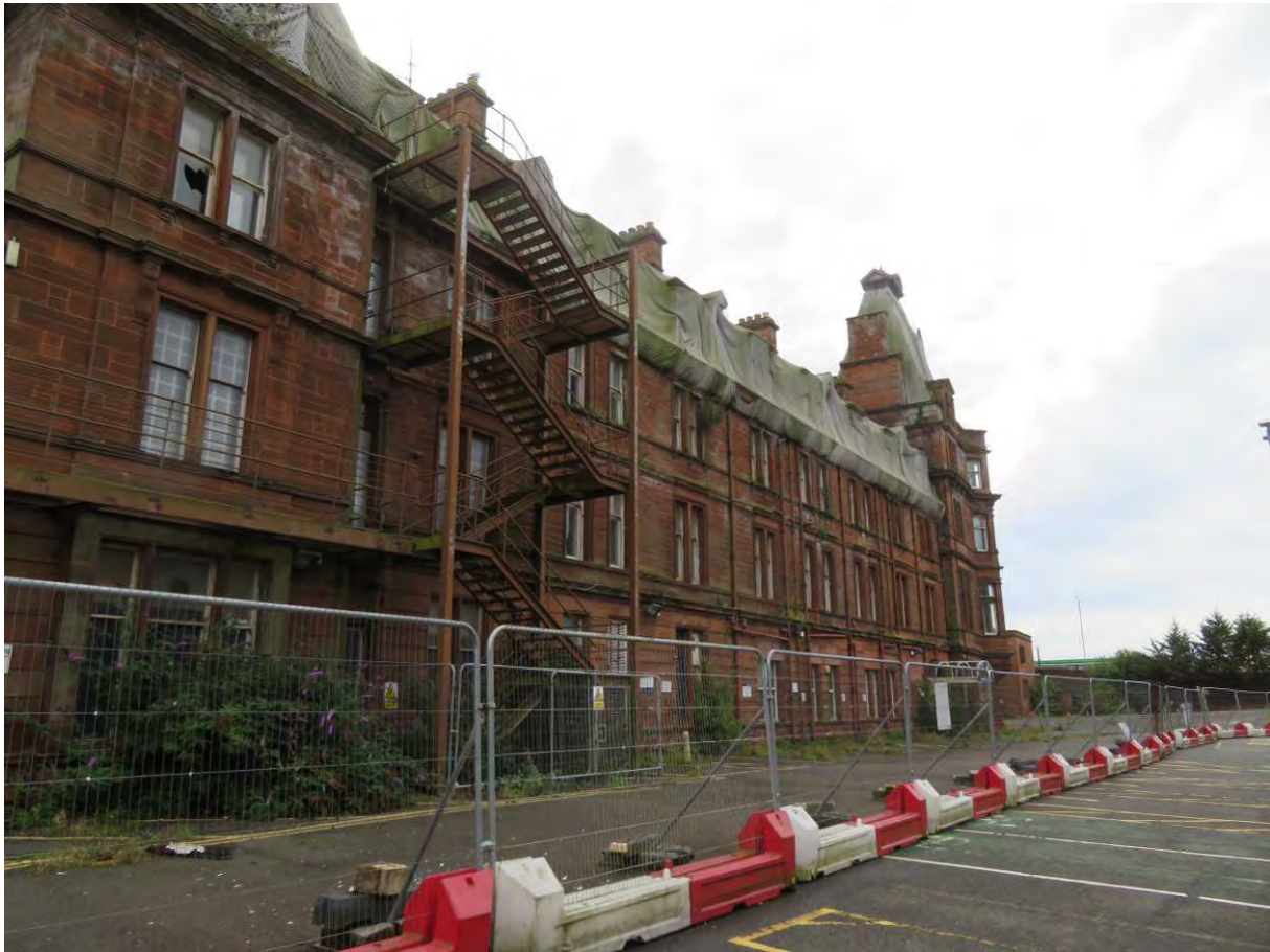
Photograph 1: North range west elevation
