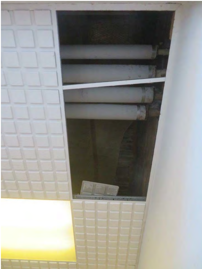
Photograph 101: Suspended ceilings in Scot Rail offices and Ticket Office
