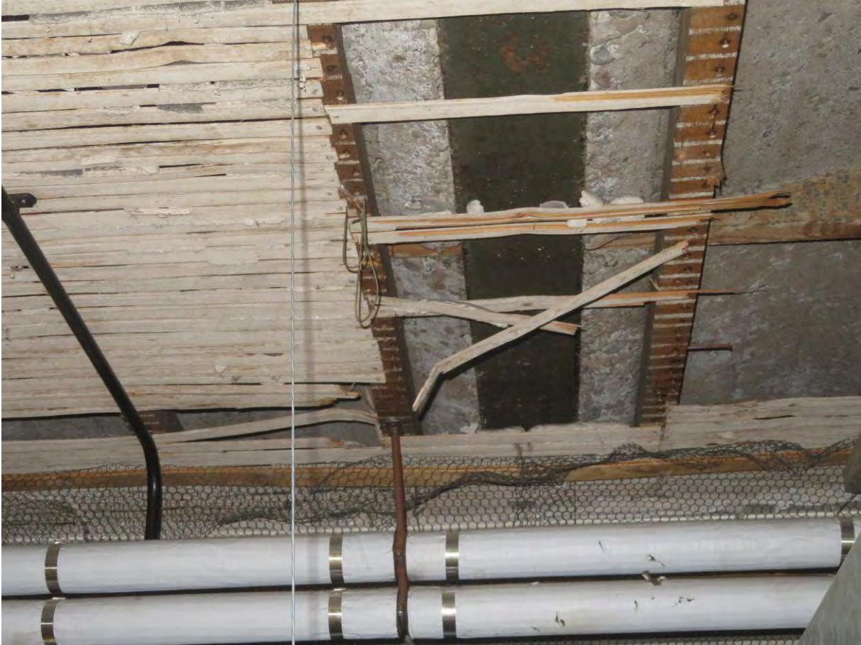
Photograph 102: Original ceilings seen above with iron joists and concrete jack arches
