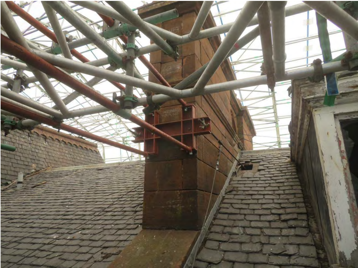
Photograph 13: Restraint arrangement using chimneys and then tying back to main scaffold
