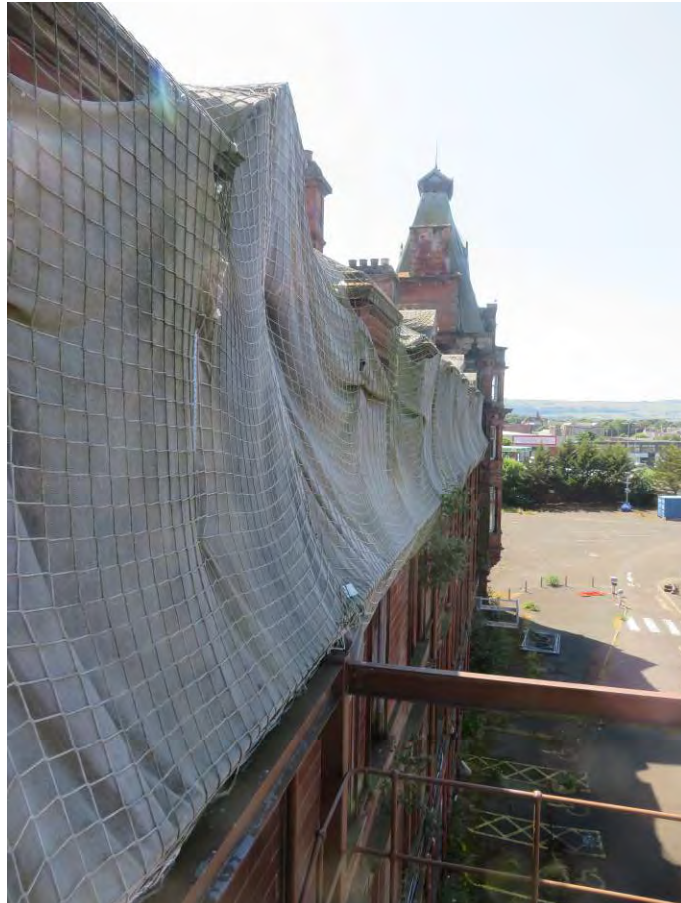
Photograph 94: Sheet covering to west elevation of north range as seen from fire escape stair
