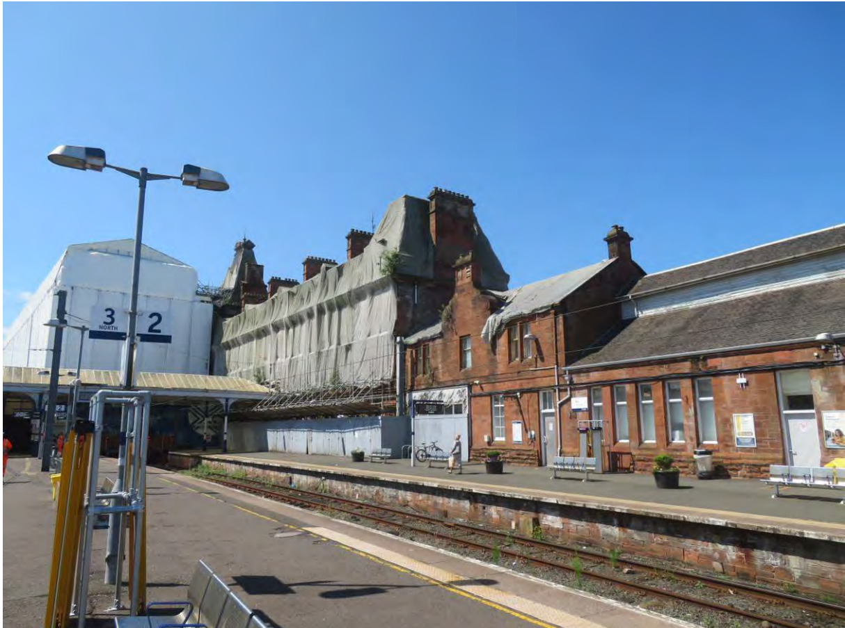
Photograph 4: North range east elevation with secondary buildings to north
