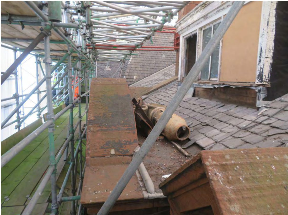
Photograph 33: Flat gutter below dormer
