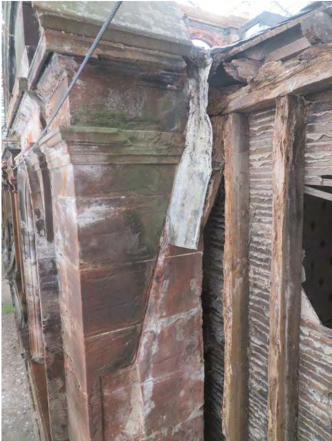
Photograph 26: Dormer to east elevation where structure fully exposed
