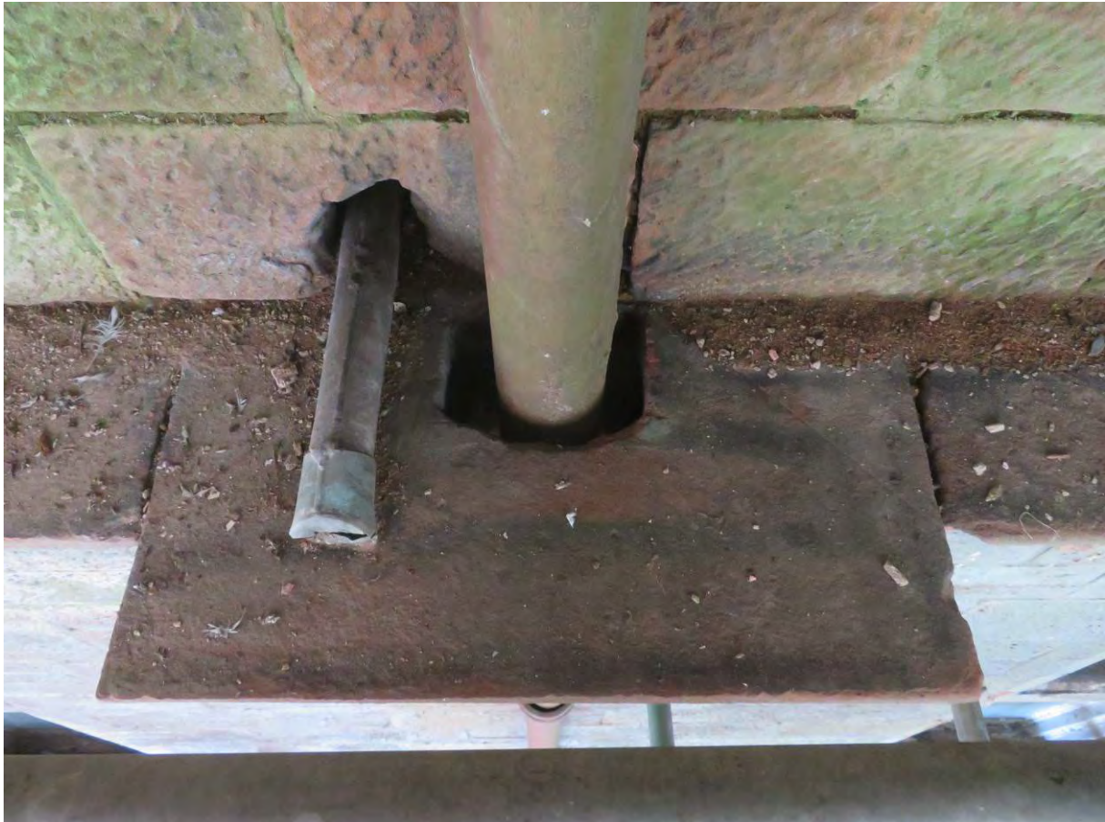
Photograph 46: Top of stone hopper
