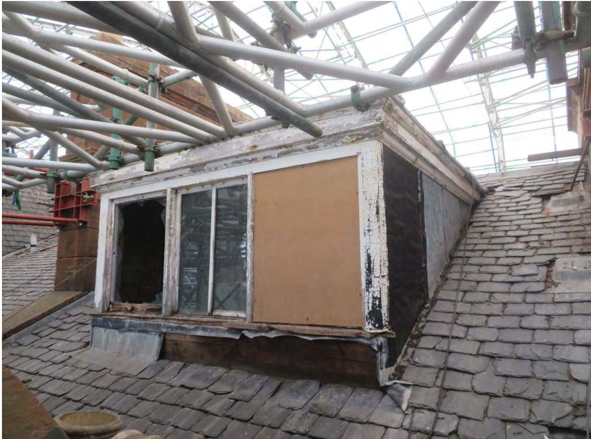
Photograph 32: Added dormer to the west elevation above lift area
