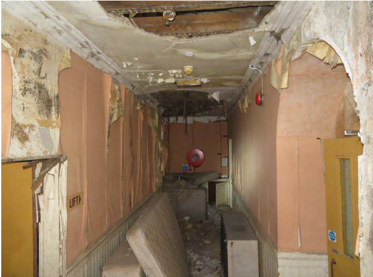
Photograph 74: Part view of ceiling with joists in foreground still sound
