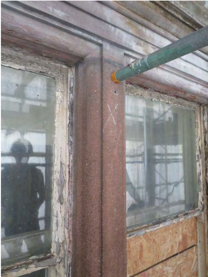
Photograph 49: Apparent coloured pre-cast concrete mullion
