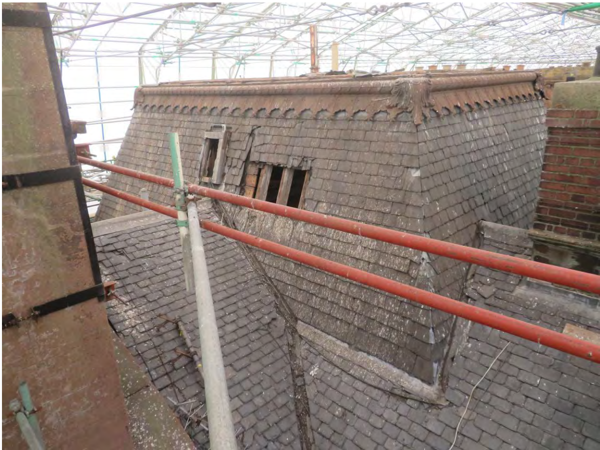
Photograph 71: Tower roof to south end of South Range
