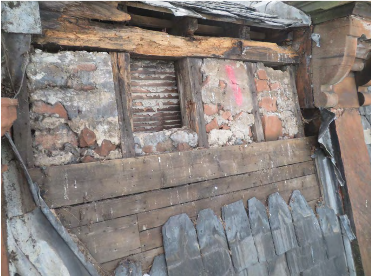
Photograph 30: Eaves detail to east elevation
