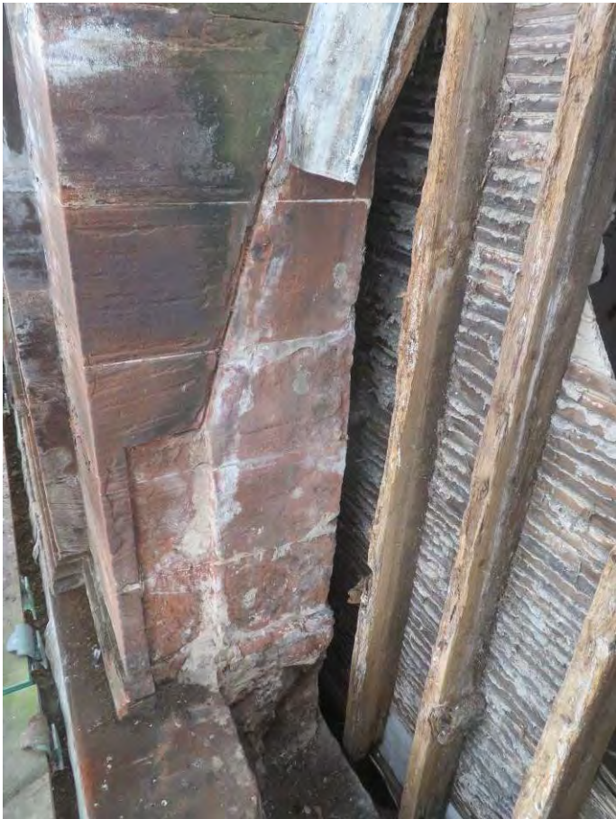
Photograph 27: Dormer to east elevation where structure fully exposed
