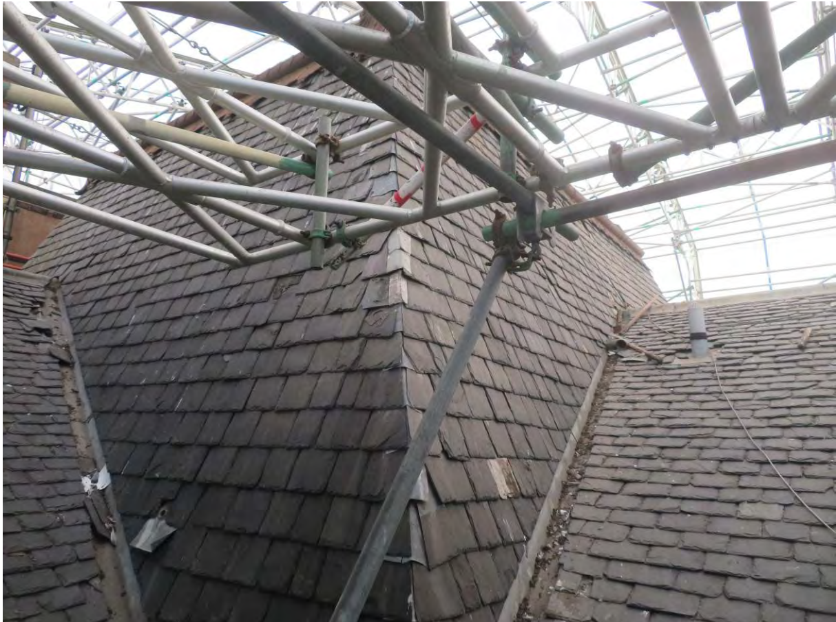
Photograph 72: North tower roof to Southern Range
