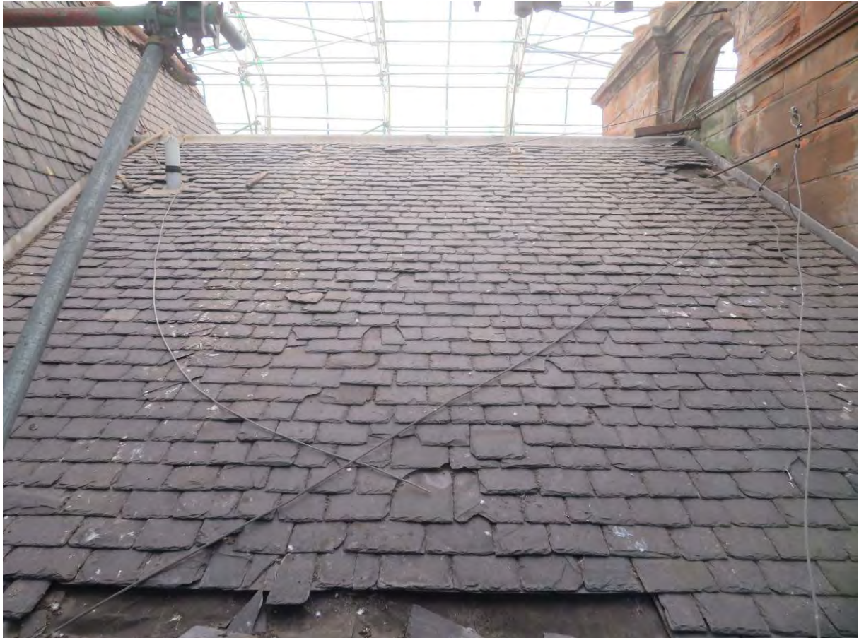
Photograph 16: Roof covering to south range west elevation
