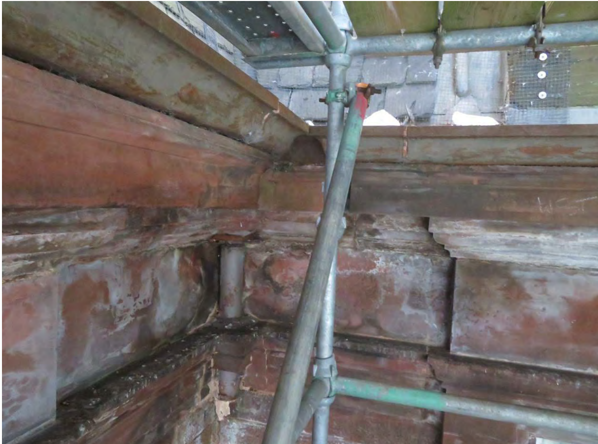
Photograph 60: North end of west elevation at junction with dog-leg
