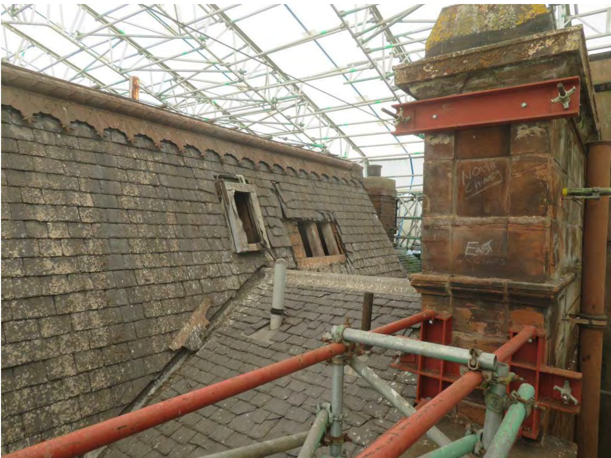
Photograph 14: Restraint arrangement using chimneys and then tying back to main scaffold
