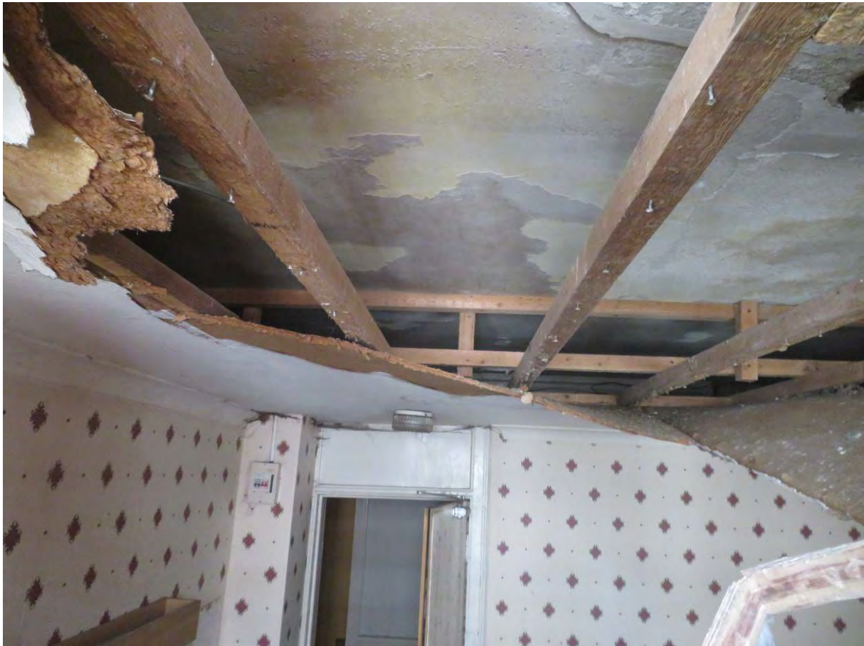
Photograph 75: Suspended ceiling below earlier ceiling above and in reasonable condition
