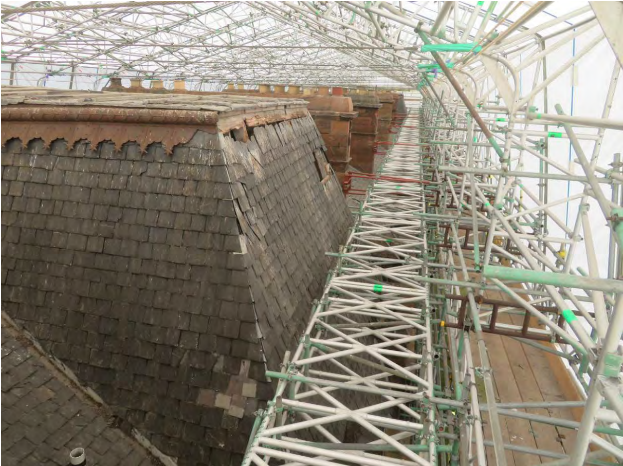
Photograph 8: High level scaffold as seen over South range
