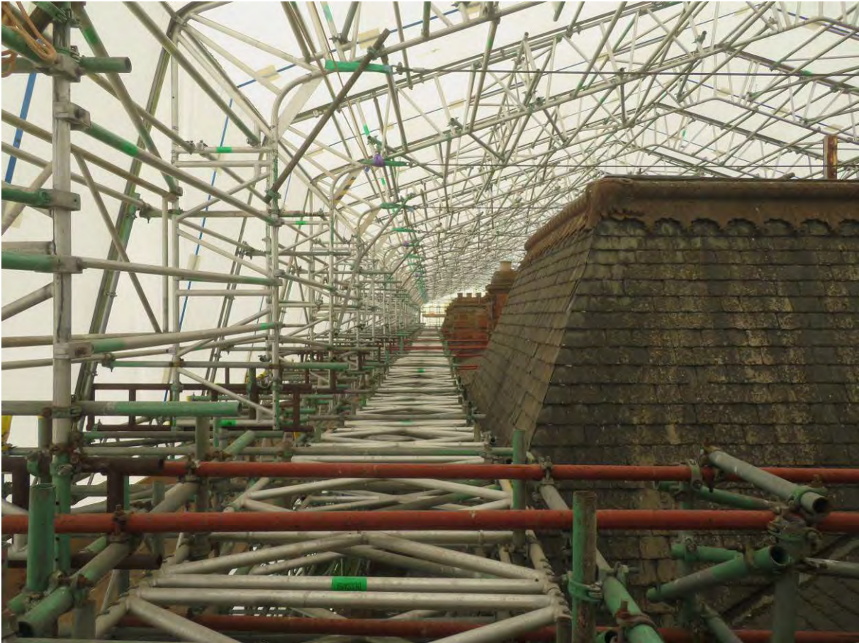
Photograph 10: High level scaffold as seen over South range
