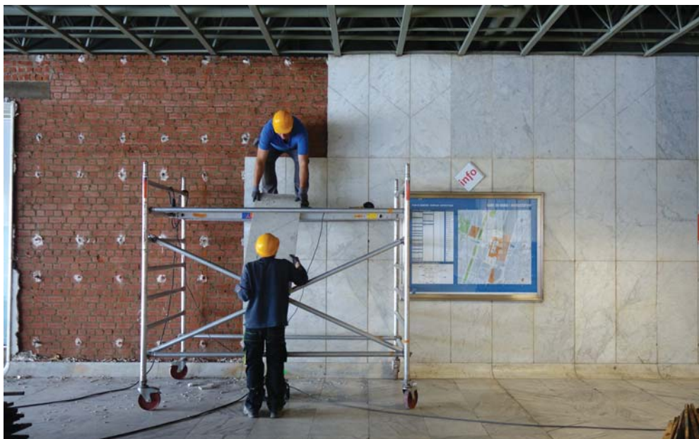
Deconstruction of a building by Belgian coop RotorDC that works to deconstruct rather than demolish buildings and find new markets for salvaged materials (Credit: RotorDC)
