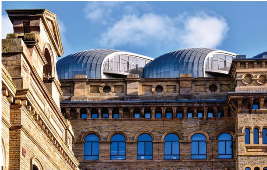
Striking view of the roof pods against the silhouette of the building's many original classical architectural details (Credit: DMA)
