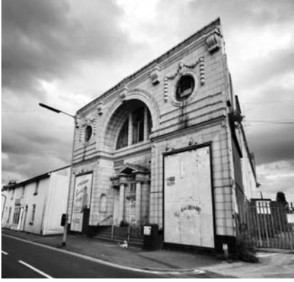
The striking triumphal arch frontage of the Sandonia Cinema, Stafford. The cinema was built in 1920 and is characterised by a distinctive white faience facade (Credit: SUF)
